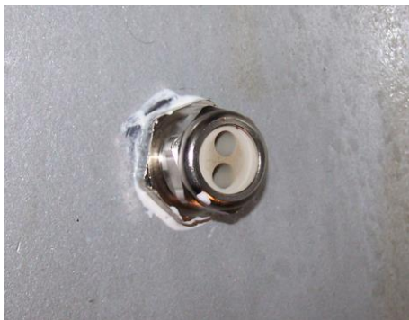
Fig. 24: Cable gland type B
